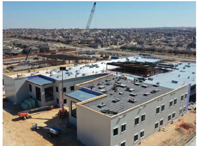
Roofing at Section 5
