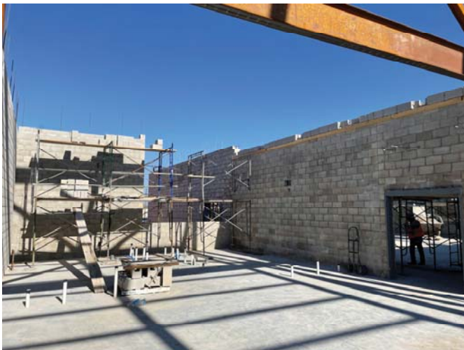
CMU Walls at Section 1
