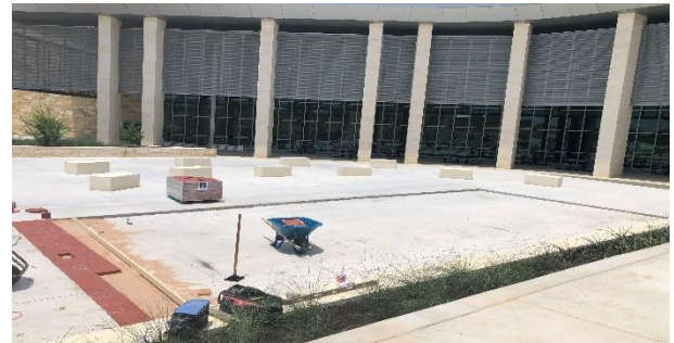
Installing Donor Pavers
