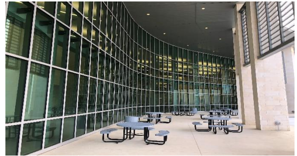
Installed Tables in Area J Courtyard
