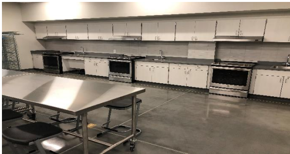
Installed Appliances in Culinary Kitchen
