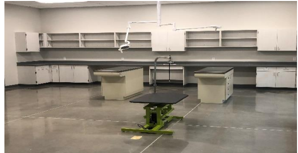
Installed Vet Tech Equipment
