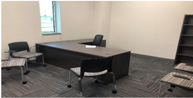
Installing Office Furniture
