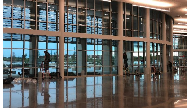
Installing Resistant Film in Area J Windows
