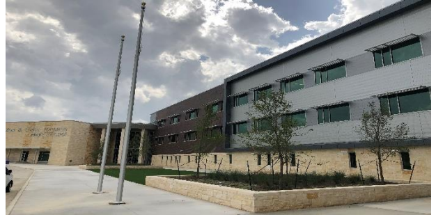
Installed Flag Poles
