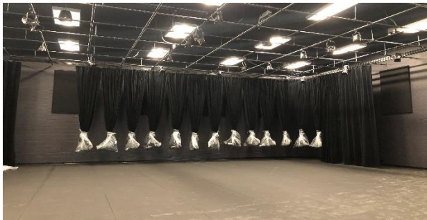
Installing Curtains at Black Box
