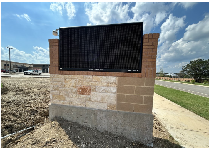
Monument Sign Installed
