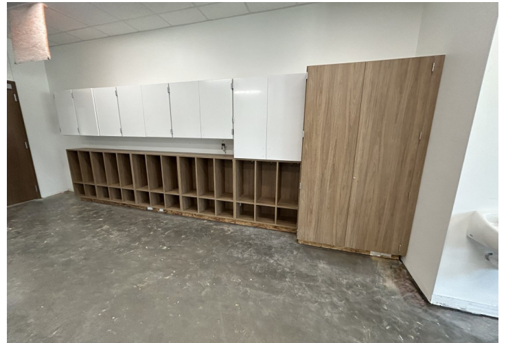
Millwork Installation at Level 1 Areas A and B
