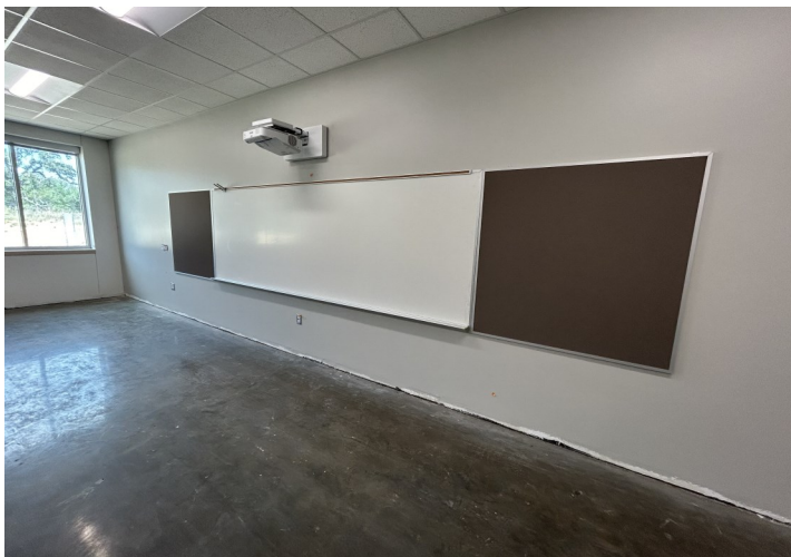
Projectors and Tackboards Installed at Levels 1 and 2
