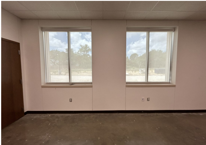
Installation of Window Shades at Levels 1 and 2
