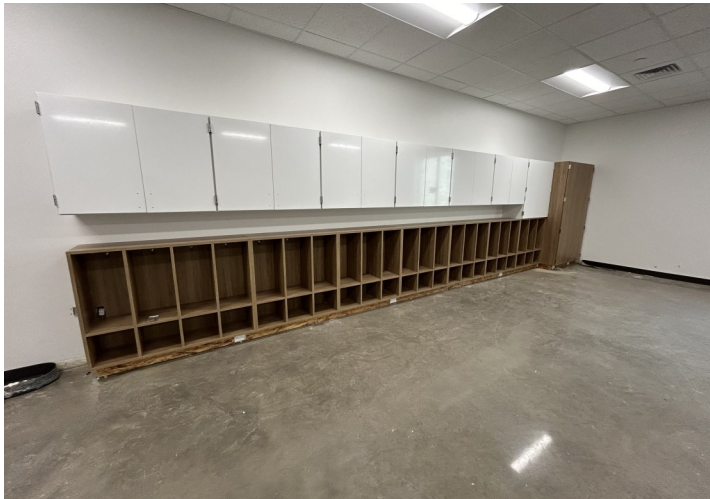
Continued Millwork Installation at Level 2 Areas B, C, and D
