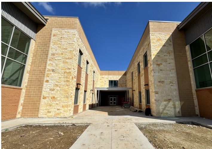
Concrete Pours at North Sidewalks
