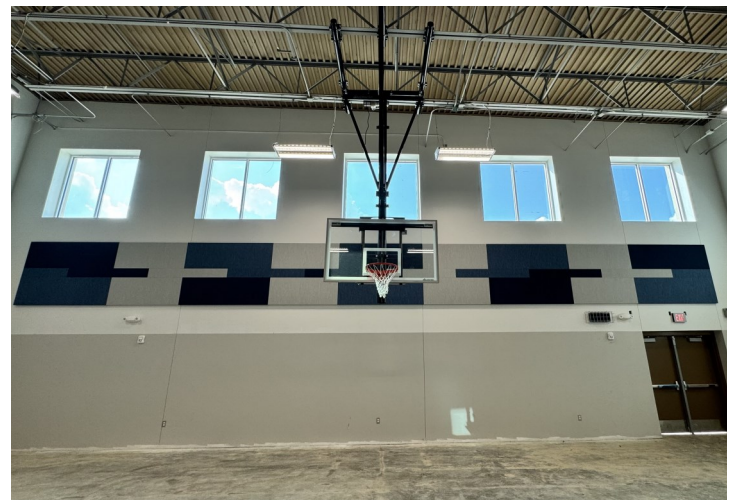
Installation of Basketball Goals
