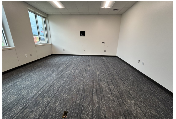
Wall Base and Carpet Tile on Level 1 and Level 2
