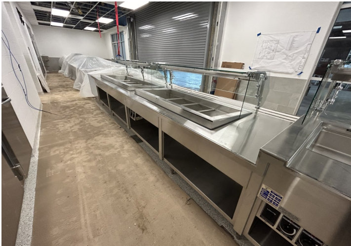
Serving Line Counters and Coiling Door Installed
