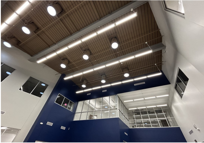
Installation of Linear Fixtures
