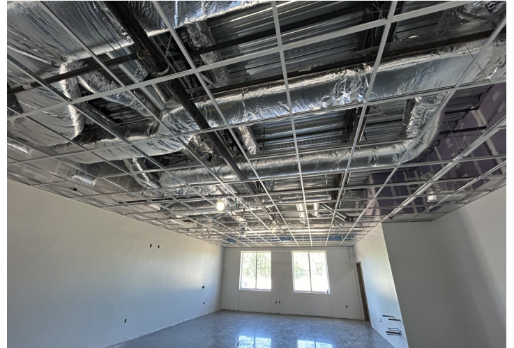
Ceiling Grid at Level 1 Areas A, B, C and D
