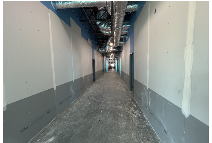
Tape and Float at Level 2 Areas C and D
