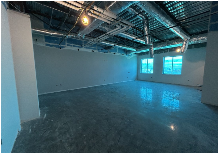
Interior Paint at Level 1 Areas C and D
