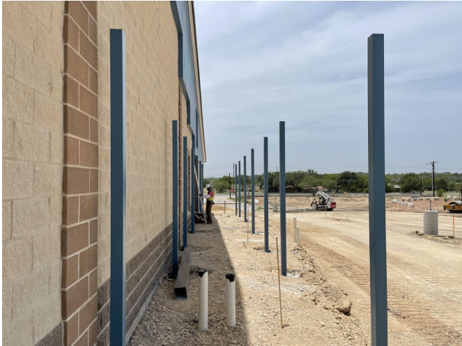
Walkway Coverings North Elevation Area A
