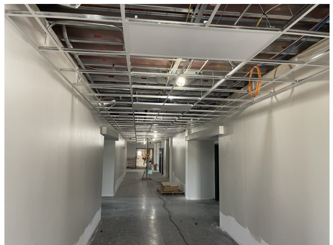
Ceiling Grid/ Light Fixtures Area A Corridors
