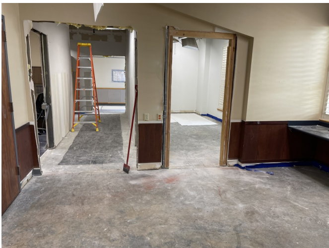
Carpet Demo Existing Admin Area
