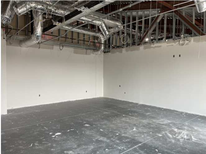
First Coat Paint Area A
