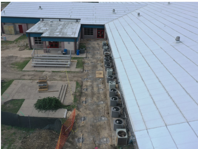
Canopy Pier Concrete
