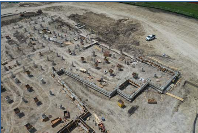
Section 3 Grade Beams
