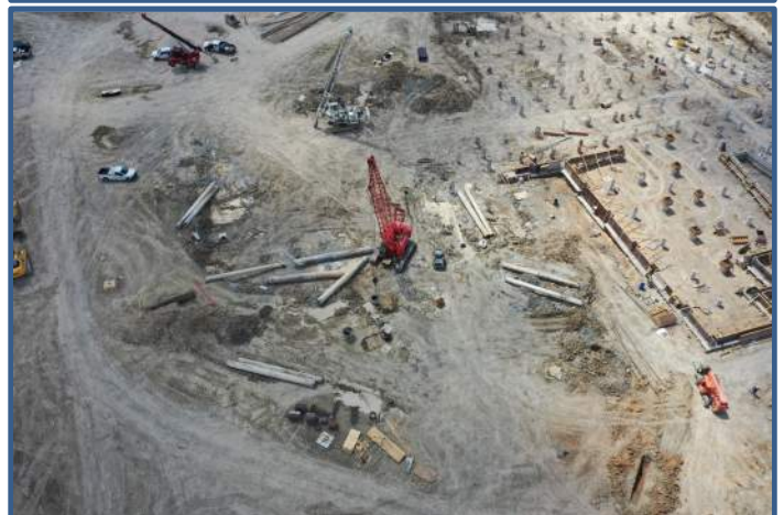
Section 1 Pier Drilling
