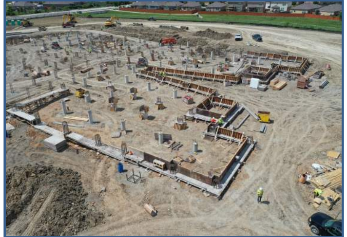
Section 3 Form Work
