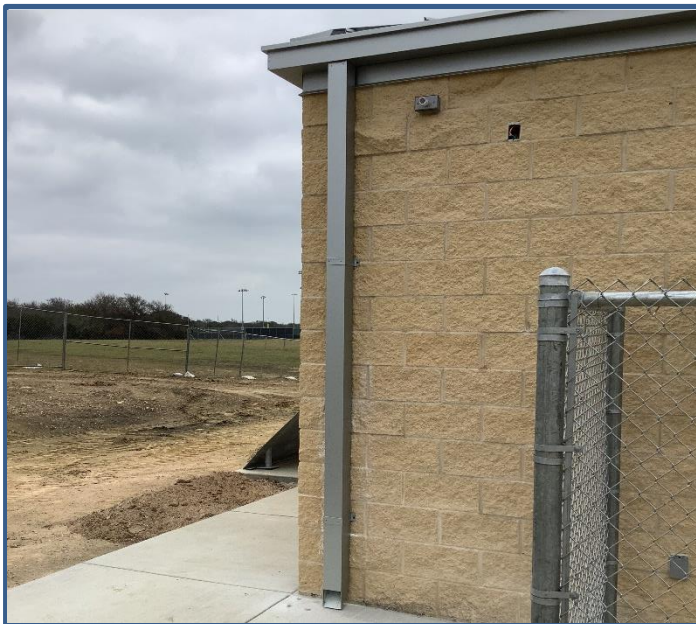
Gutters and Downspouts Complete
