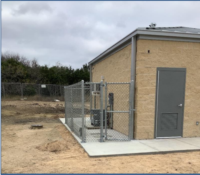
Fence Complete around Transformer Pad
