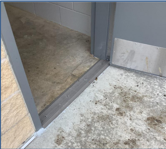
Thresholds Installed at Entrances
