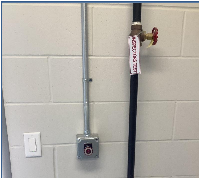
Emergency Push Button in Progress
