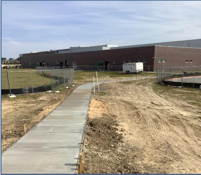
Sidewalk Concrete Poured
