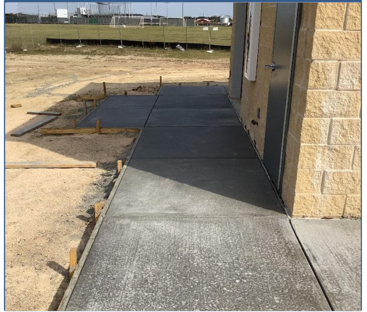
Sidewalk around Building
