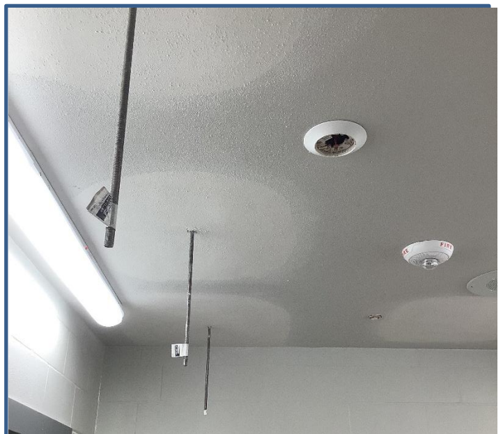
Hangers for Mesh Ceiling Installed
