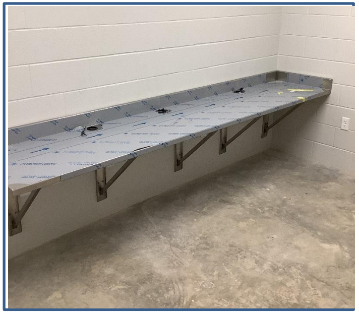
Metal Countertop Installed
