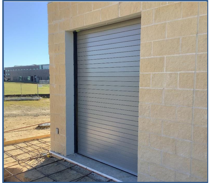
Overhead Coiling Door Installed
