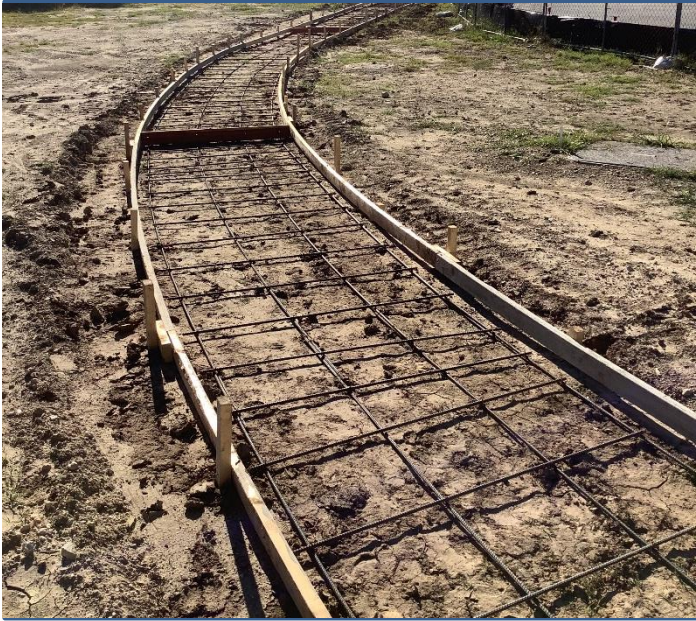
Sidewalk Formed and Rebar Installed
