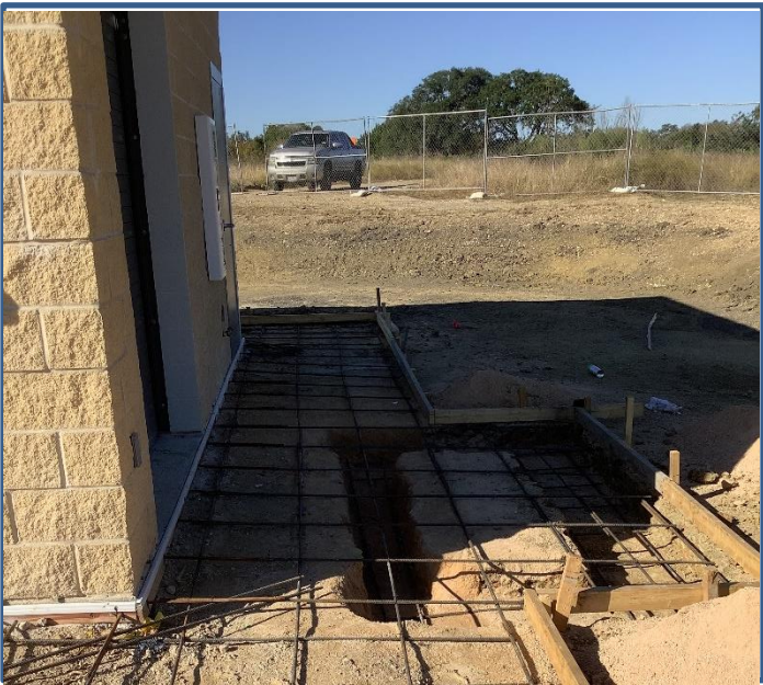
Sidewalk Around Building Formed
