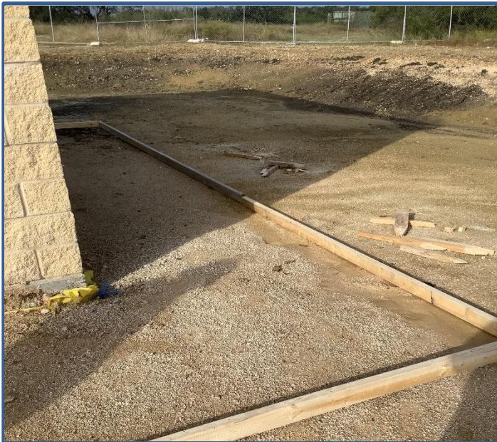
Building Sidewalk Formed
